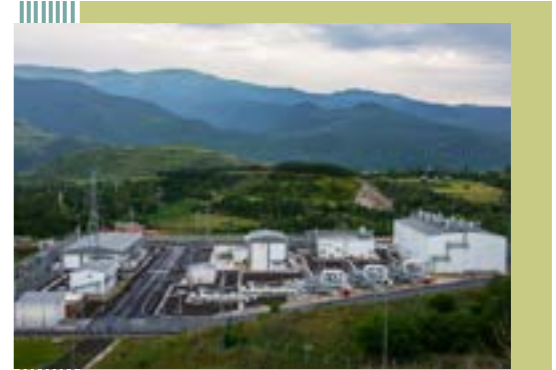
Metering Station (MS1), Ardahan
