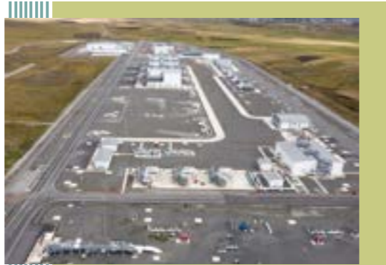
Compressor Station (CS1), Ardahan
