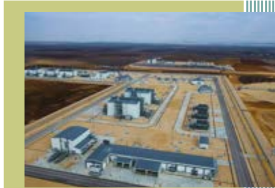
Compressor and Metering Stations (CS5-MS2), Eskişehir
