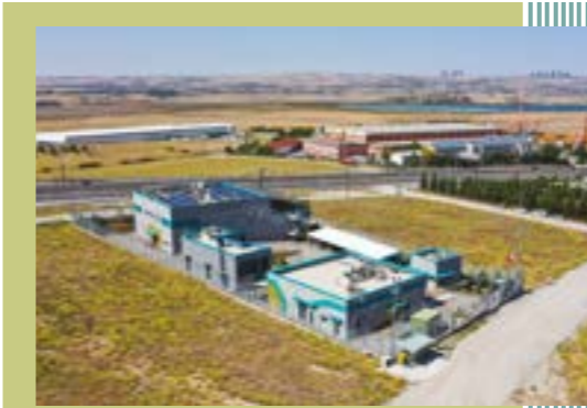
Main Control Center (MCC), Ankara
