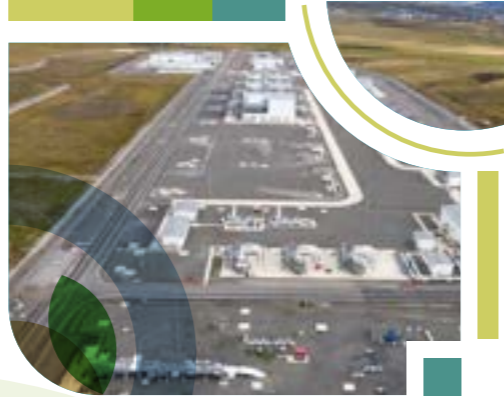
Compressor Station (CS-1) Ardahan
