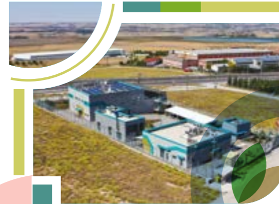
Main Control Center (MCC) Ankara
