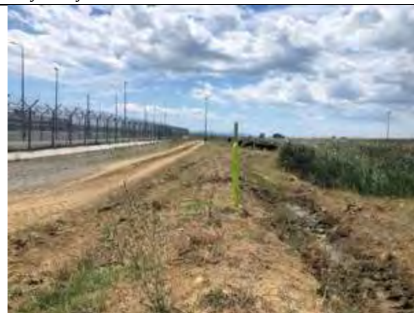
Poor reinstatement Lot 4 MS 4, TAP exit point (issue already known of TANAP)
