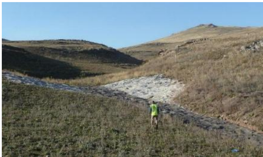
Figure 12: New scour protection solution at RVX4-5101
