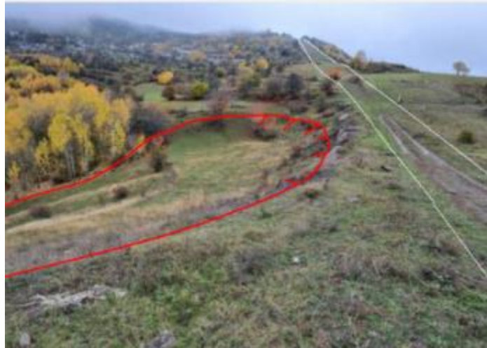
Figure 8: Active landslide adjacent to the ridge at ~ KP16
