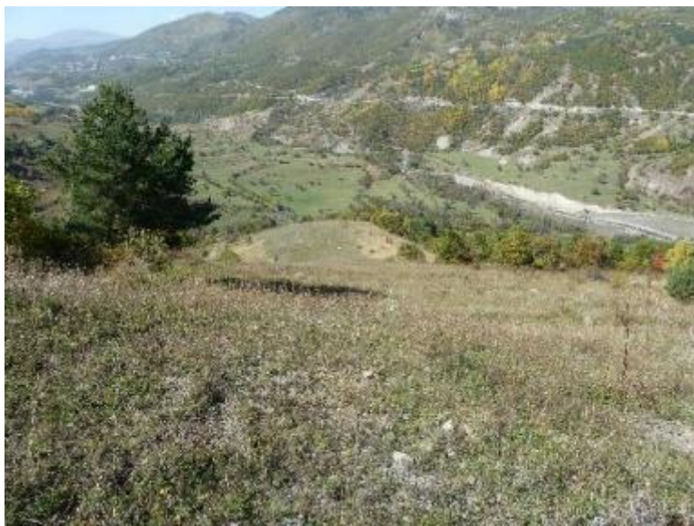
Figure 11: Well stabilised slope at KP14+900
