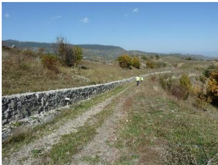
Figure 10: RoW along the Ridge at KP16+442
