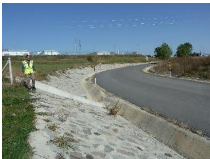
Figure 14: New drainage channel at MS1
