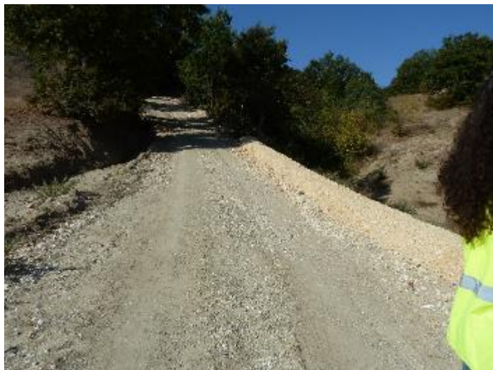
Figure 12: Berm at the top of the riverbank to divert surface water run-off
