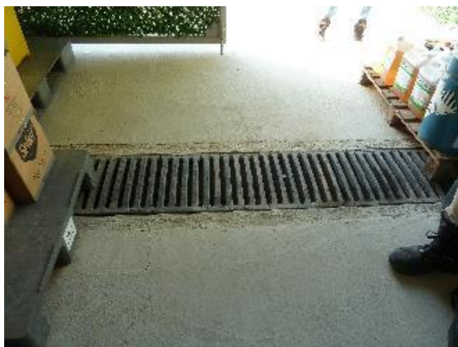
Figure 22: Closed drainage
