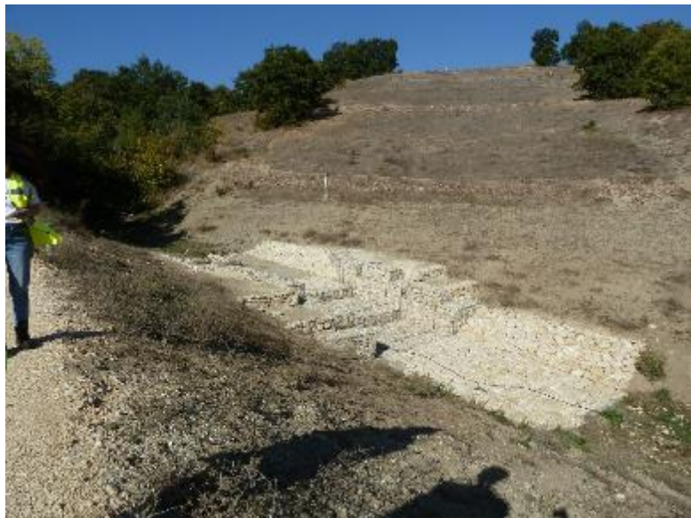
Figure 11: Gabion wall/rip rap to mitigate scour at RVX4-0699
