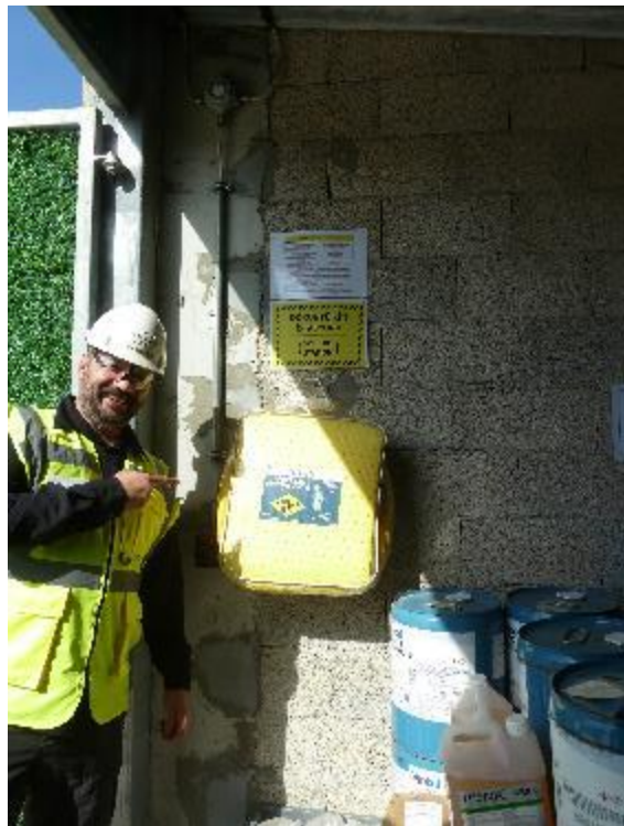
Figure 21: Provision of spill kits within the hazardous materials storage facility
