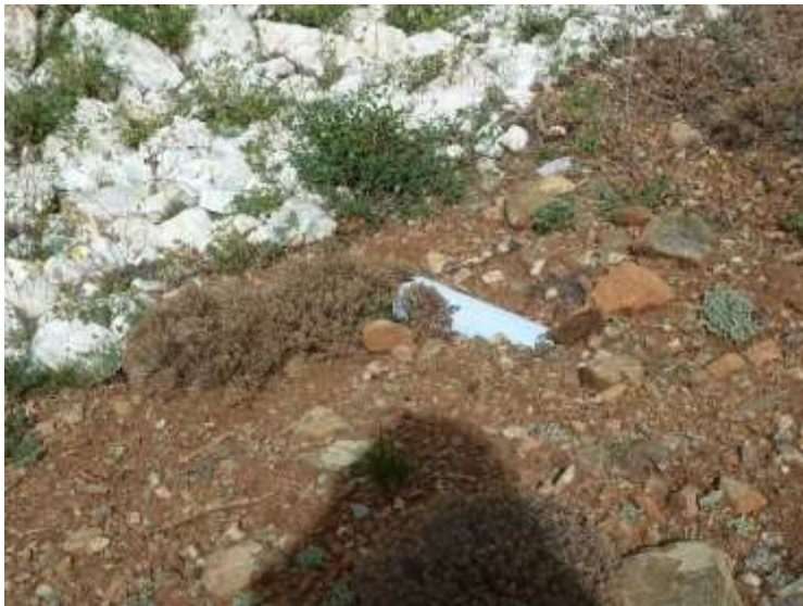
Figure 2.10: Pipe discharging from the trench to a permanent slope breaker
