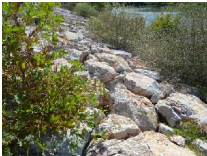
Figure 2.6: Rip Rap at KP 1661 in good condition
