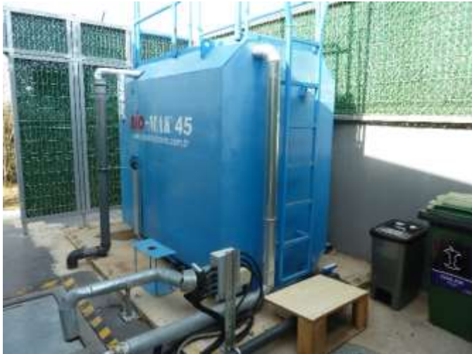
Figure 2.20: Biological wastewater treatment plant at the MCC
