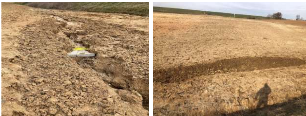
Figure 2.13: Concrete slab exposed and gully backfilled
