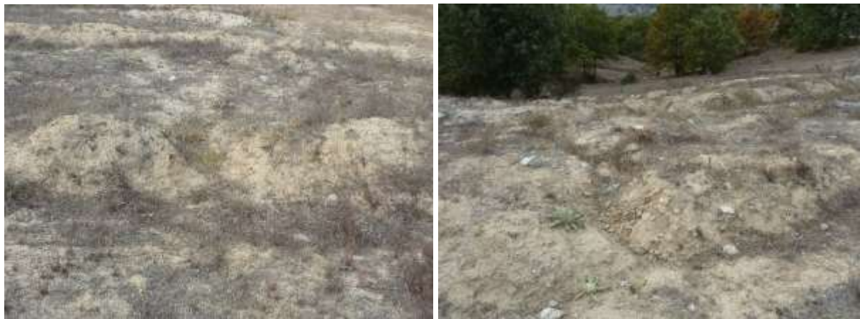
Figure 2.8: Breaches of slope breakers and gullies forming
