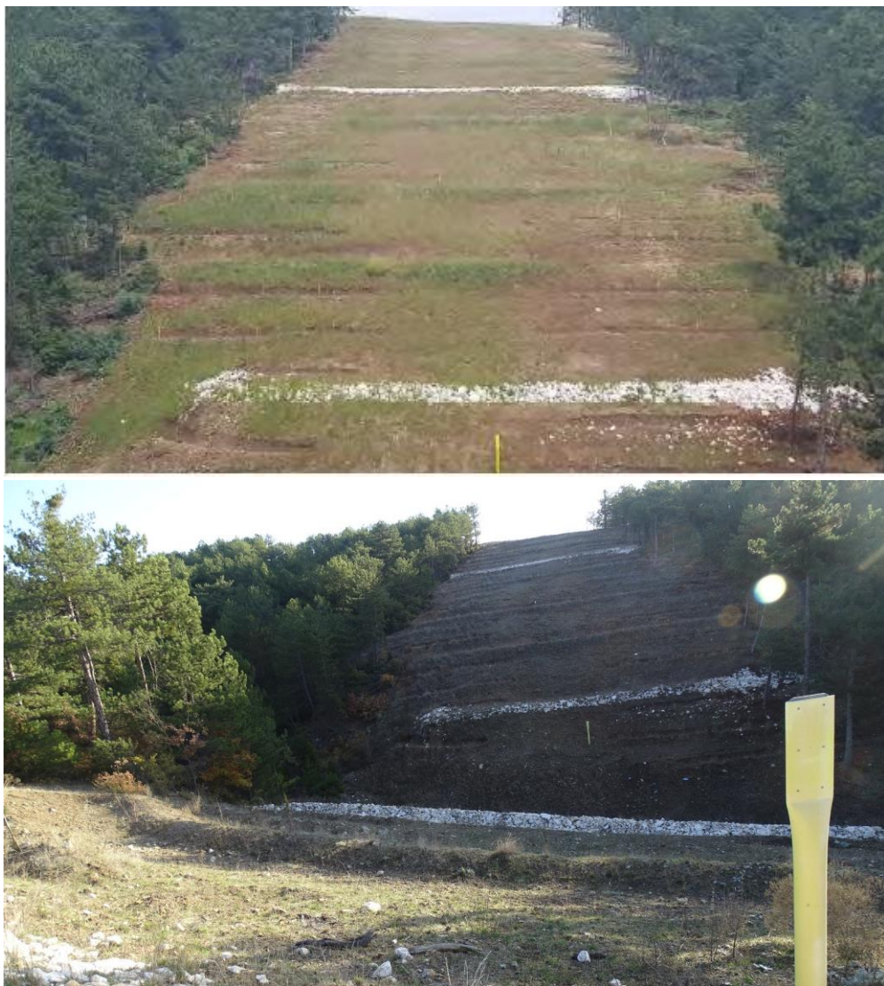
Figure 2.12: Migration of rocks from the slope breaker at KP 1504+910 (2020 / 2021)
