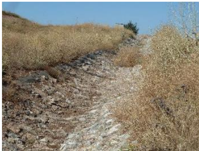
Figure 2.13 Permanent flood diversion channel
