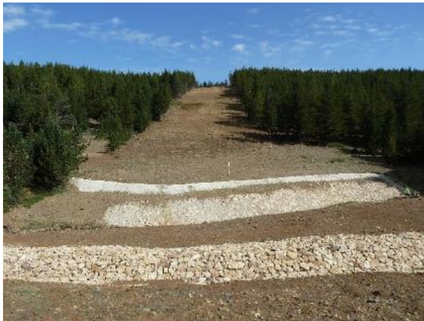
Figure 2.11 Additional permanent berm and slope breaker at KP 617+207
