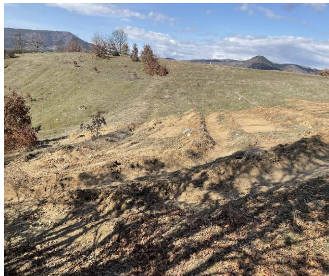
Figure 2.9 Repairs made at KP 1518+302
