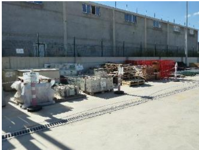
Figure 2.18 External materials storage area at CS3
